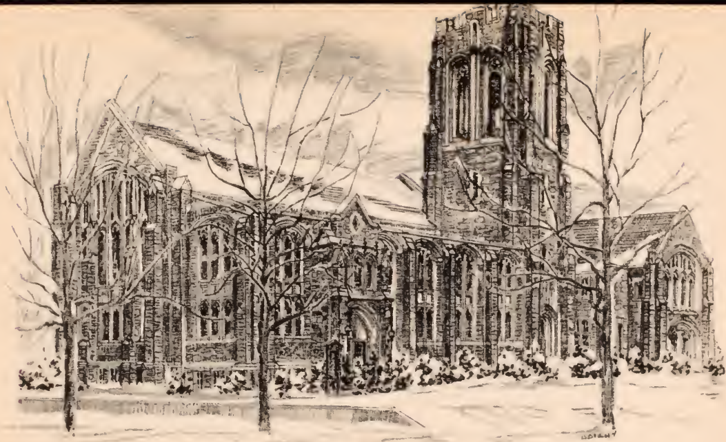
COLLINGSWOOD PRESBYTERIAN CHURCH, COLLINGSWOOD, N. J.
